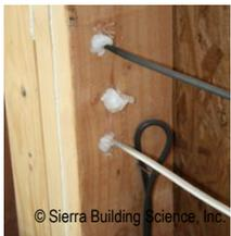
**Sealing the Air Barrier:** Seal all gaps around windows, doors, behind tubs and showers, etc. Caulk or seal all gaps in the air barrier greater than 1/8” with foam.
