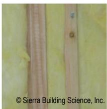
**Correctly Sized Batts:** Batt insulation should be cut to fit snugly at the sides and ends without gaps or buckling. It should not double over or be compressed and should be friction fit to cavities, or otherwise supported. Batt insulation should be split to fit around wiring or plumbing, and trimmed to fit around junction boxes.
