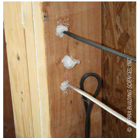
Sealing the Air Barrier
