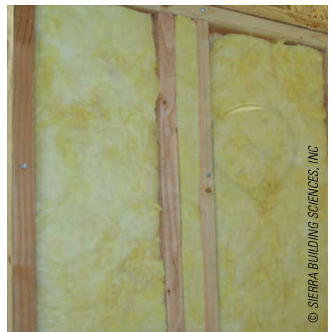
Correctly Sized Batts
