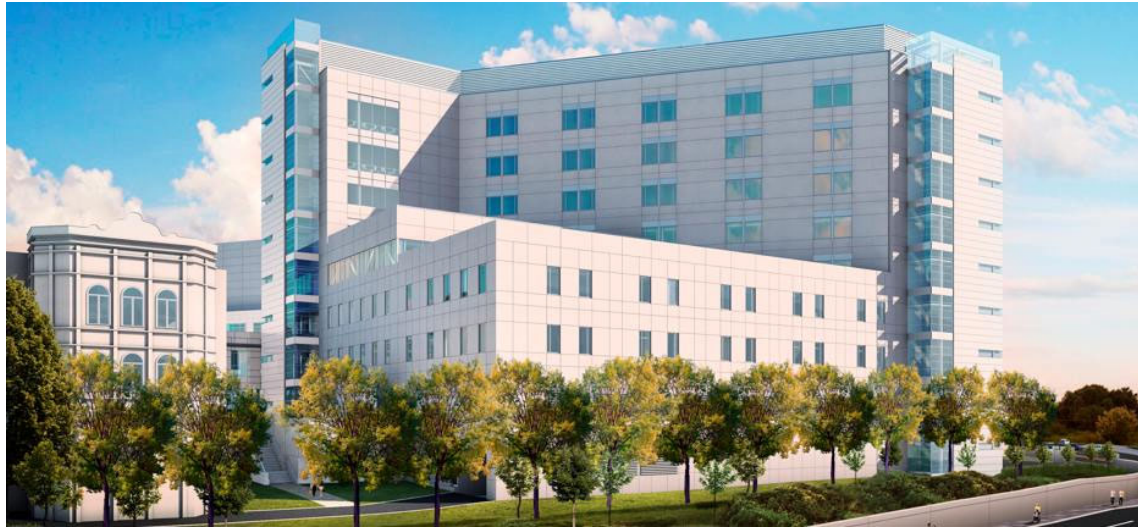
Highland Hospital, Oakland CA (picture courtesy of Ted Tiffany, Guttman & Blaevoet Consulting Engineers)
